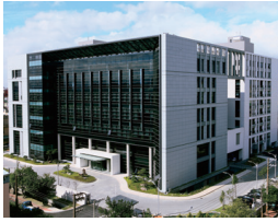
Taoyuan Technology Center (Green Building)
